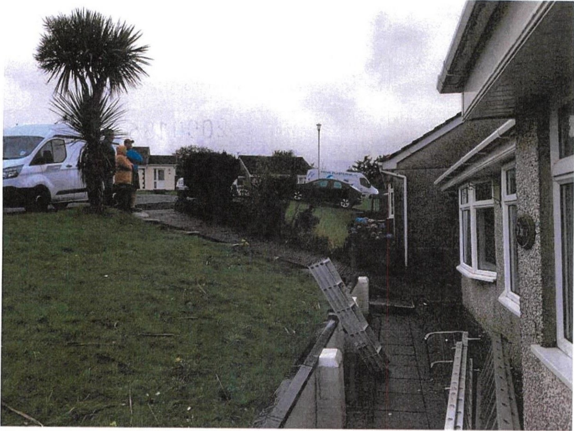
Photograph demonstrating the excessive steepness of the existing driveway
